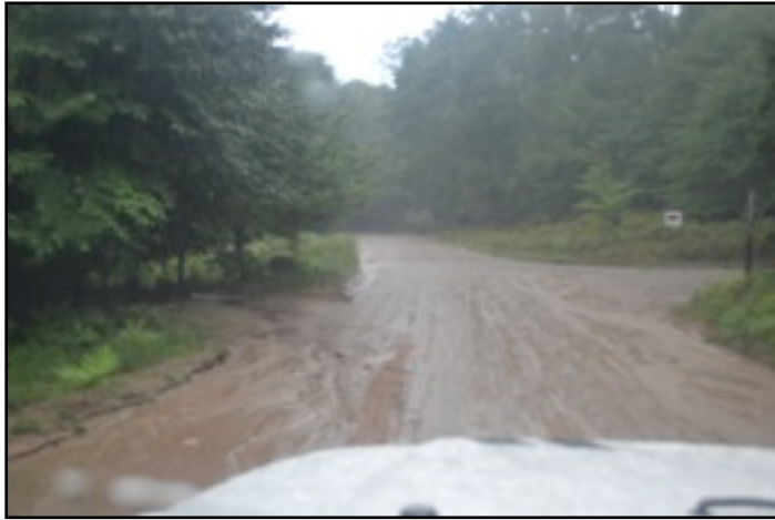
Fox Den at Lookout Trail with soaker pit on left, erosion leading into the pit.
